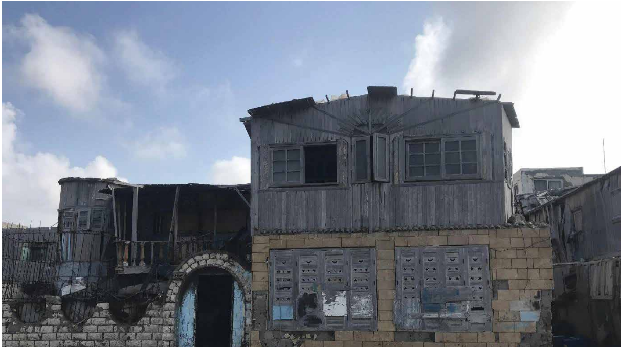
Fig. 2 The lighthouse residences (photo: Y. Osman)
