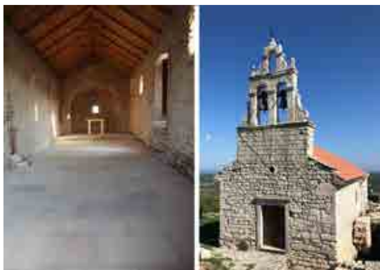
Fig. 25. New paving in the interior and the restored bell-gable on the façade of the present-day Orthodox parish church of Sts Joachim and Ann at Bribir (photo: A. Milošević)
