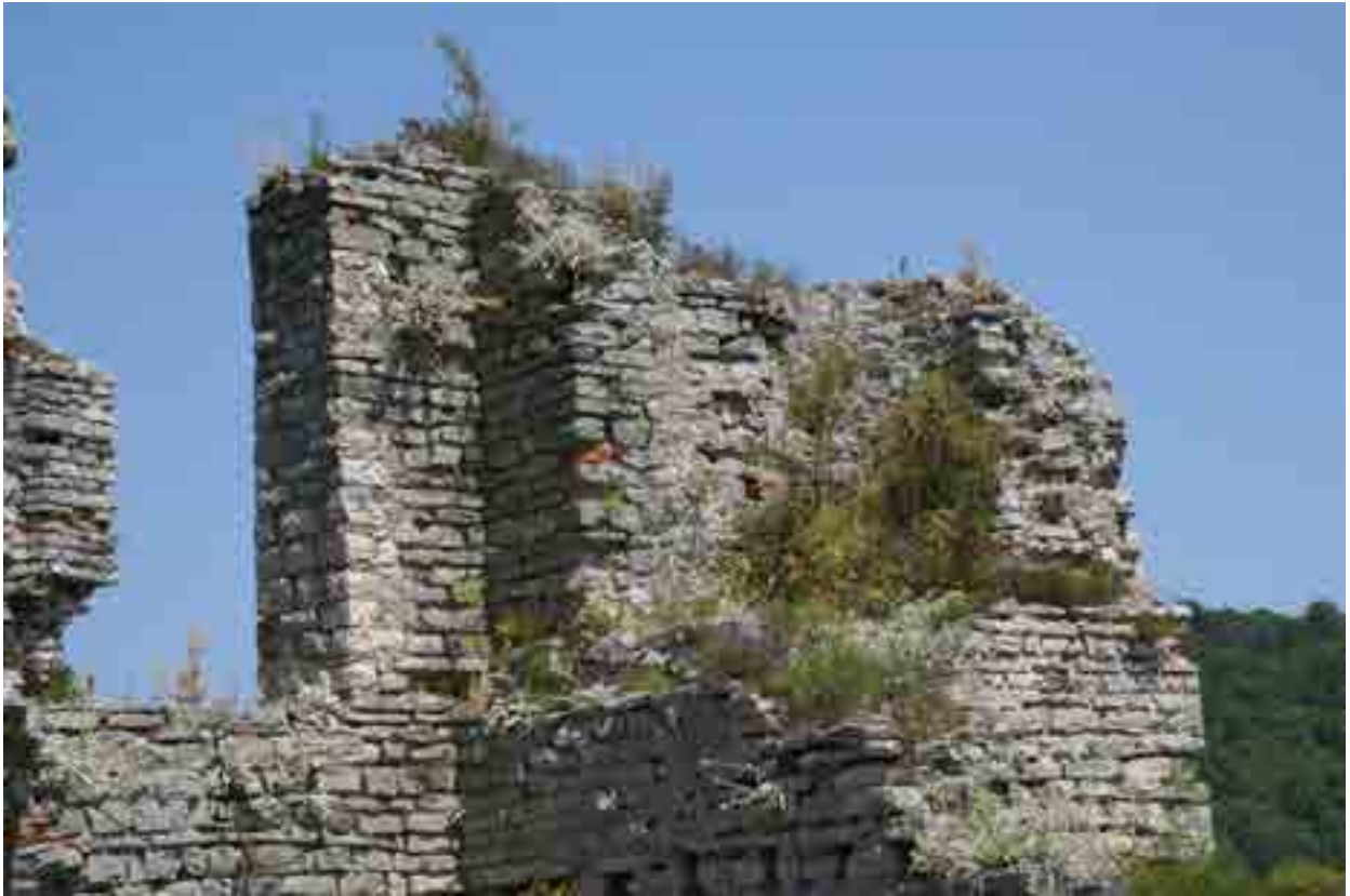
Fig. 7. Remains of a buttress niche on the palace first floor (photo: Ž. Peković, 2010)
