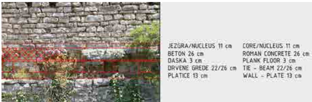
Fig. 11. Reconstruction of the floor structure cross-section based on the triclinium wall indentations, Ž. Peković, 2011
