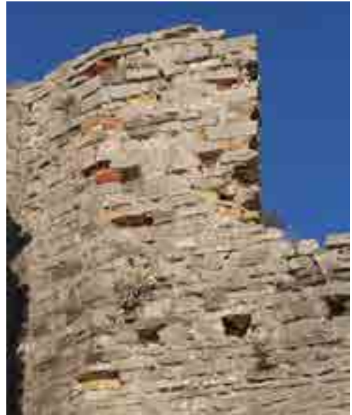
Fig. 9. Remains of lateral frames of the upper floor window in the tower (photo: Ž. Peković, 2010)
