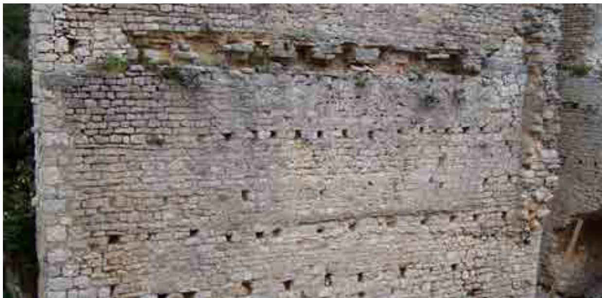
Fig. 10. The audience hall lateral walls with remains of floor structure indentations (photo: Ž. Peković, 2011)
