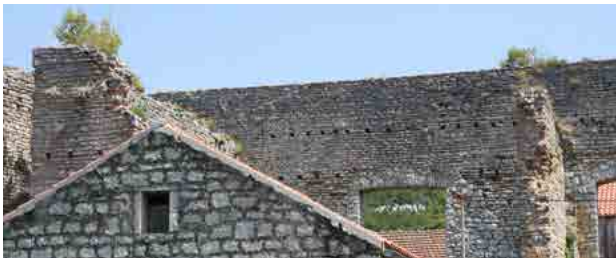
Fig. 12. Remains of roof structure on the lateral wall of the audience hall (photo: Ž. Peković, 2010)
