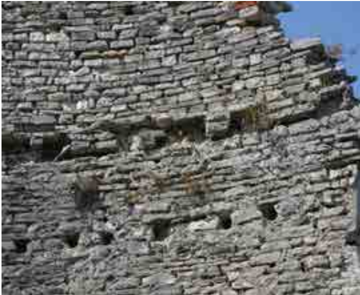
Fig. 8. Indentations of the wooden floor structure in the tower (photo: Ž. Peković, 2010)
