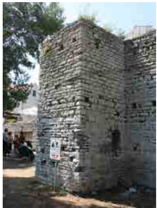
Fig. 6. The façade buttress with a sanitary niche window (photo: Ž. Peković, 2010)
