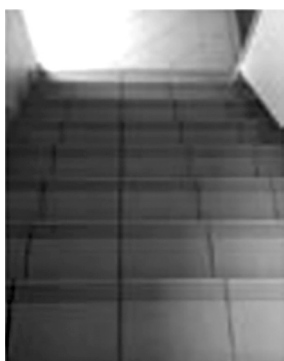
PICTURE 1 Contrasting orientation lines on the stairs and hallway of the school Source: Kozmus (2019: 56)
