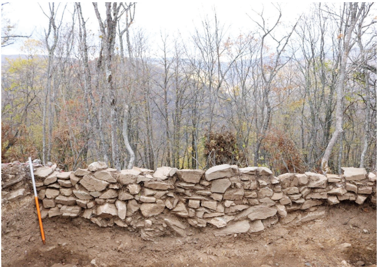
FIGURES 12 AND 13 Northern perimeter wall of the fortress of Marec (Z. RAMA, 2018) SLIKE 12. I 13. Sjeverni zid utvrde Marec (Z. RAMA, 2018.)
