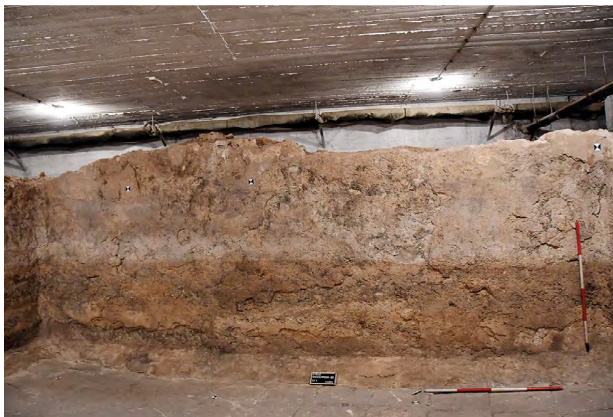
Sjeverozapadni zid vodospreme (foto: V. Glavaš) Northwestern wall of the water reservoir (photo: V. Glavaš)
