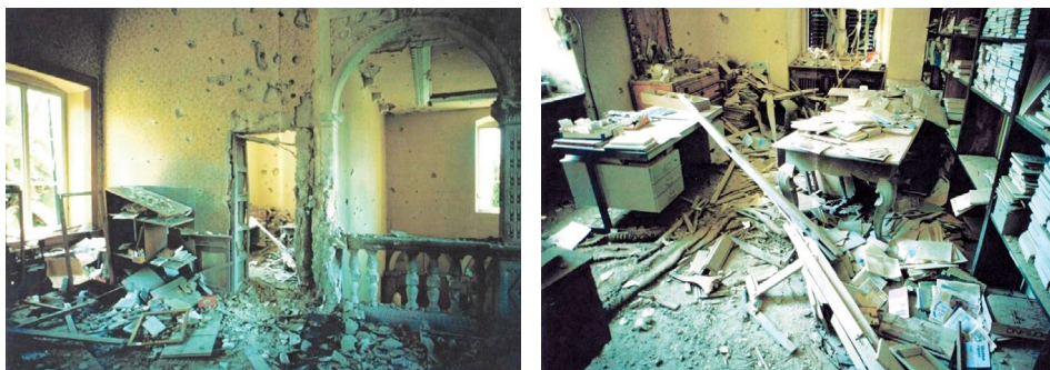
Figure 5 and 6. Damage to the first floor of the Library, June 8th, 1992 (Source: Digital photo archive of Dubrovnik Libraries)
