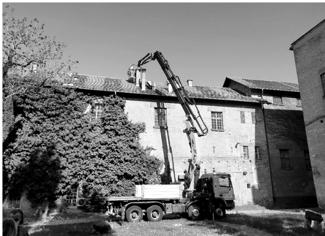
Figure 3. Pulling down the chimneys (Source: Photographic Collection of the Glyptotheque)
