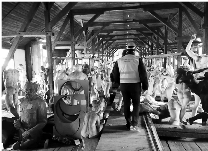
Figure 2. First inspections of the museum buildings by Civil Defence officers (Source: Photographic Collection of the Glyptotheque)
